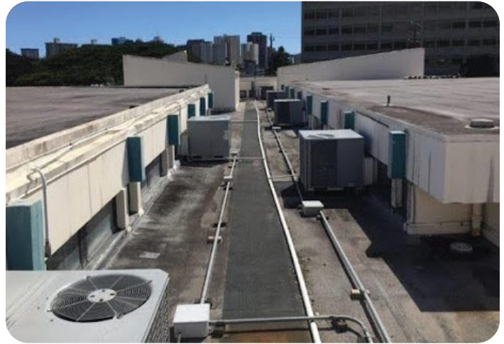
Old roof that was gutted and retrofitted in Fall 2023.
