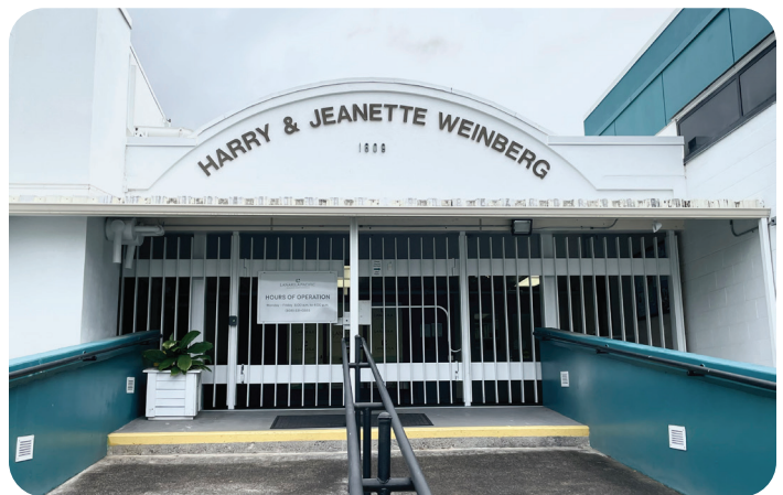
New flood barrier to be installed at the main entrance in 2024.
